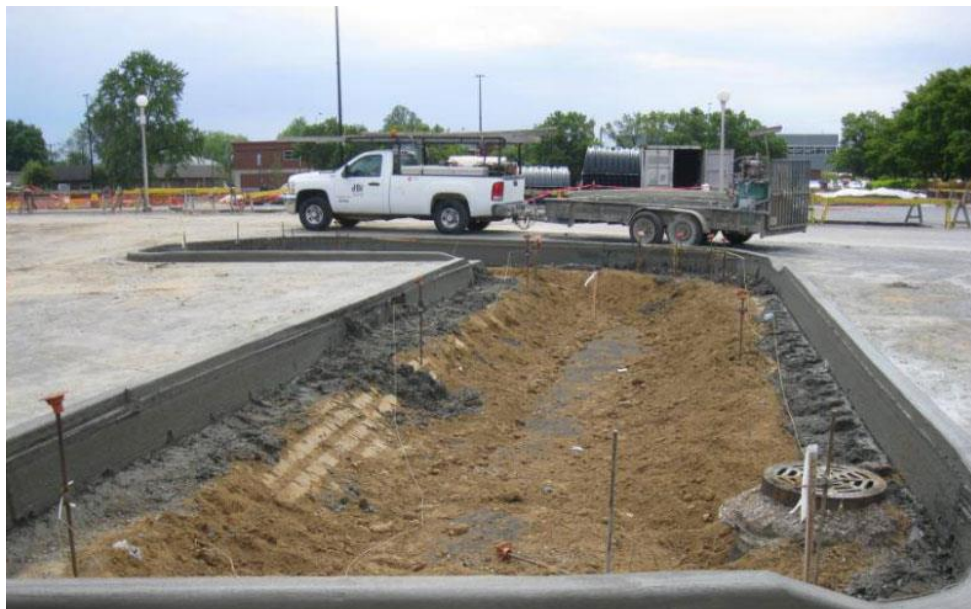
Figure 8-12: Construction of Bioretention Cell in Parking Lot, Evansville, IN (source: Indiana Office of Community & Rural Affairs)
