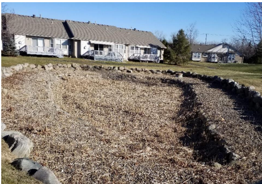
Figure 8-3: Dry Detention Basin (source: OHM Advisors)
