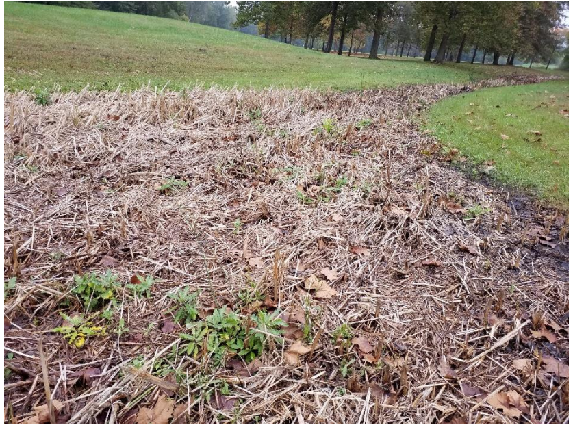
Figure 7-7: Example of a swale (source: OHM Advisors)
