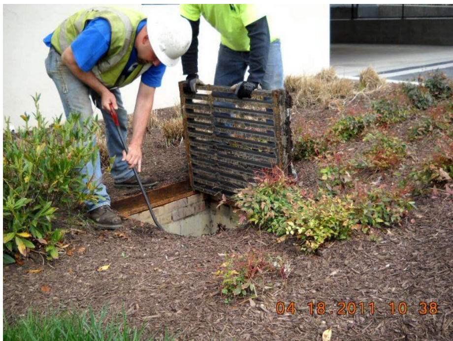
Figure 9-1: Bioretention Clean Out (source: Stormwater Maintenance Consulting)
