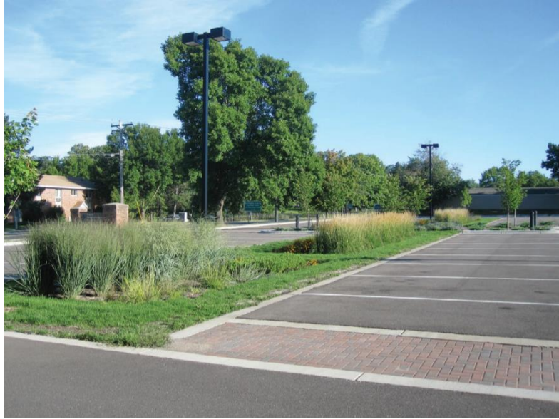
Figure 6-1: Parking lot bioretention (source: US EPA)
