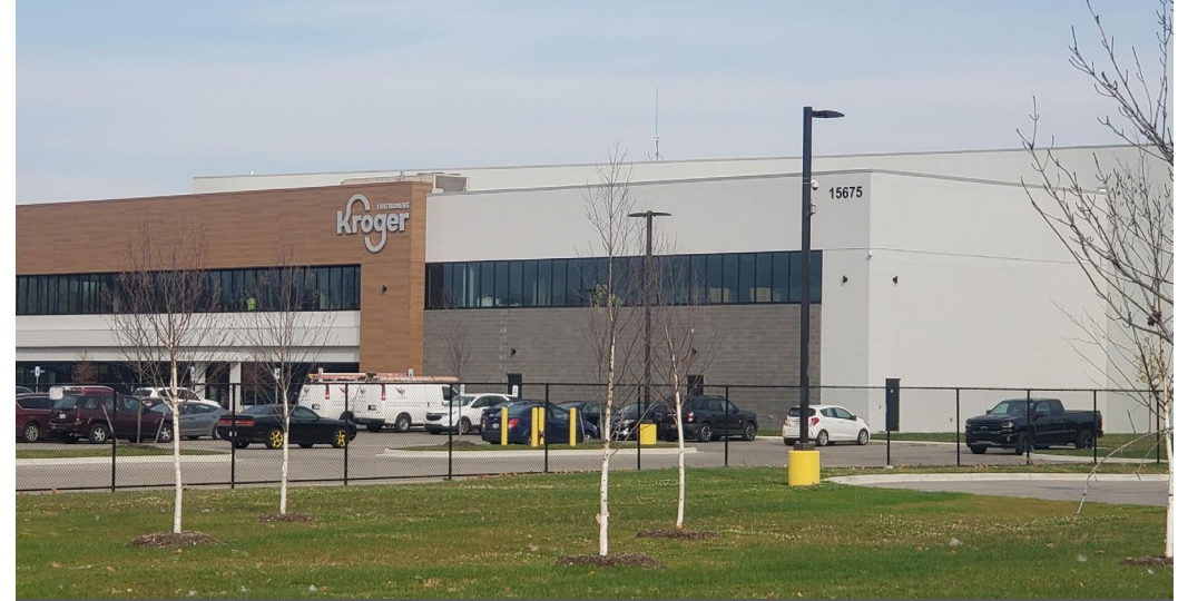
Kroger Distribution Center along Wahrman Rd
