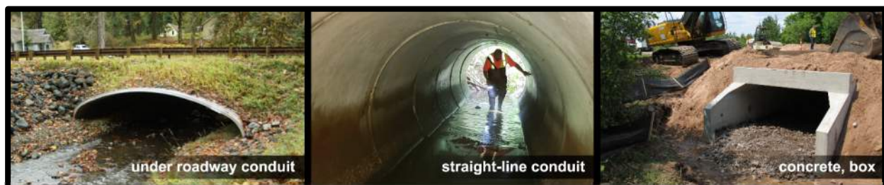
Figure B-2: Examples of culverts. Culverts allow water to pass under the roadway (left), they are straight-line conduits with no intermediate drainage structures (middle), and they come in various materials (left: metal; middle and right: concrete) and shapes (left: arch; middle: round; right: box).
